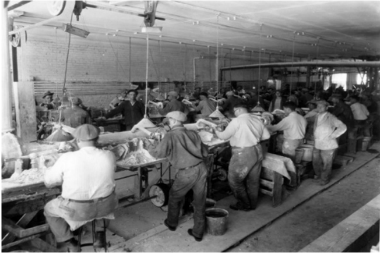
Figure 6: Conveyor belt, Cincinnati Slaughterhouse, 1870
